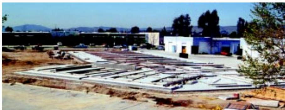
*Construction in progress (top). The walls started out horizontal (above). The walls are tilted up, hoisted in place by crane (facing page, left). The last piece of wall goes into place (facing right).*
