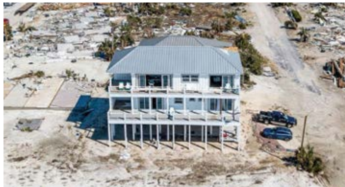
Mexico Beach, Florida, home built by Dr. Lebron Lackey with design specifications for materials and construction methods to withstand 250 mph winds.
