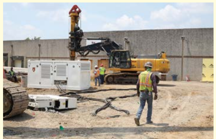
Pile-driving equipment digging for pier placement for the Discovery Center's planetarium and auditorium foundation.
