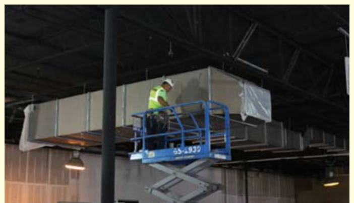
Installing air ducts and plumbing to prepare the exhibit hall.
