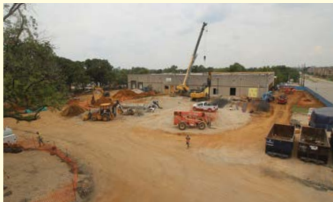
Pile-driving equipment digging for pier placement for the Discovery Center's planetarium and auditorium foundation.
