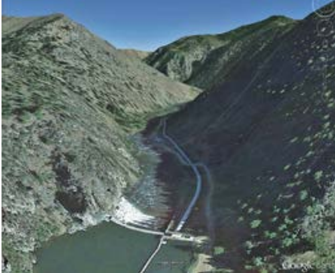
Landsat satellite image of a hydroelectric dam on the Madison River in the bottom of Bear Trap Canyon. Image: Google Earth
